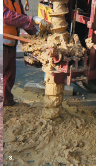
1. Measuring standing water level (Colac, Victoria); 2. Completed piezometer at a mine site (Ardlethan, NSW); 3. Hollow augering through a clay aquitard (Horsham, Victoria).
