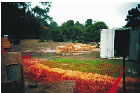
Off-site sedimentation control using bidum filter socks or hay bales.
