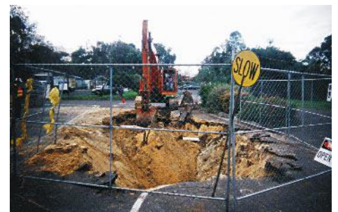
Barricading and fencing around open excavations.
