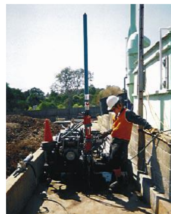
The Mark II light-weight, push-tube drilling rig in a tight spot.
