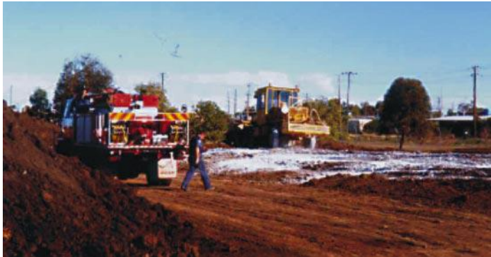
Remediation of PAH contaminated soil is promoted by aeration with soil ameliorants, cotton trash and surfactant..
