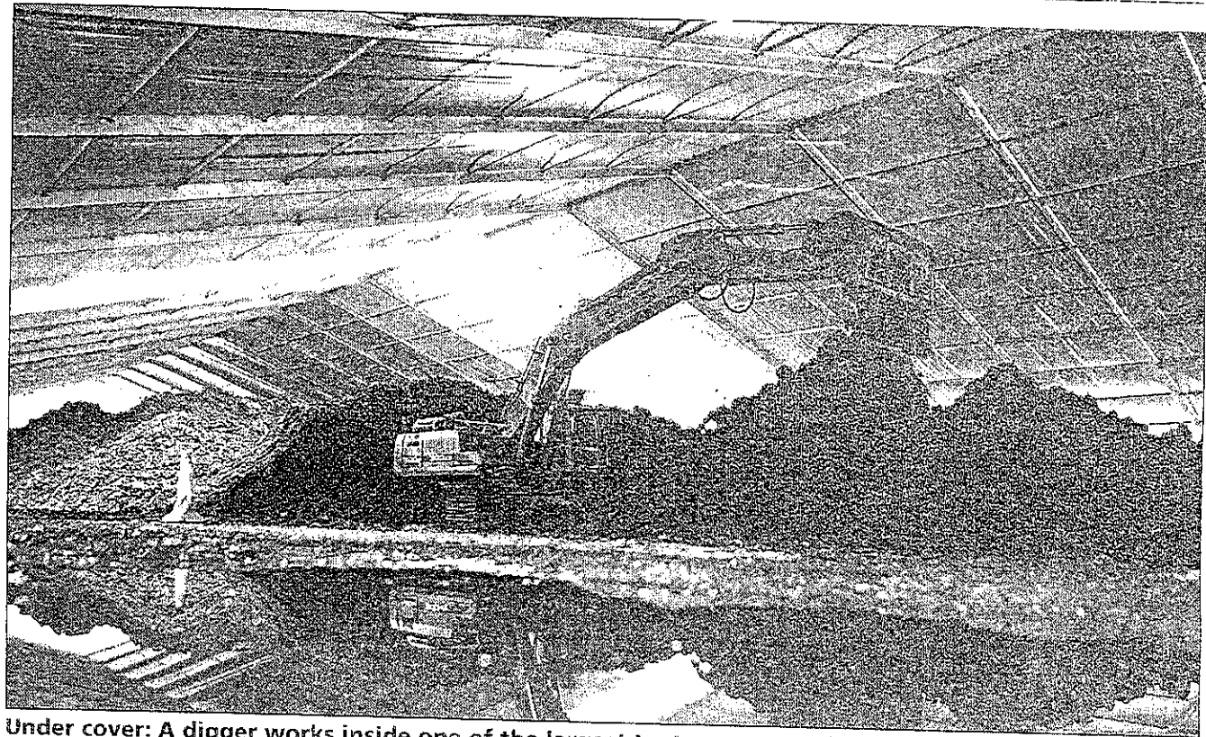
Under cover: A digger works inside one of the largest tents ever erected in Hull as part of a major environmental improvement programme at the city's former gasworks in Clough Road.
